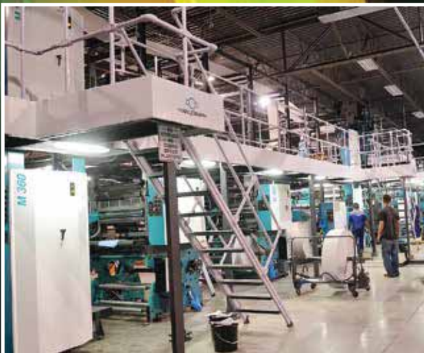
The 20-Unit M360 installed at Paxton Media, North Carolina, U.S.A.
